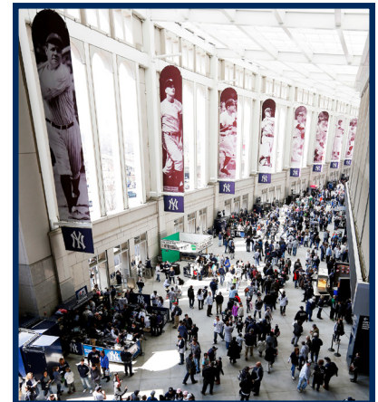
The majority of Yankee Stadium guests enter the building via the 31,000-sq.-foot Great Hall. Built with massive open-air archways that allow for ventilation, it does not require air conditioning.
