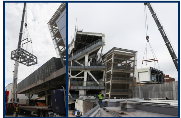
On March 4, 2024, a 550-ton, state-of-the-art, water-cooled, modular chiller plant was raised to the centerfield roof of Yankee Stadium.
