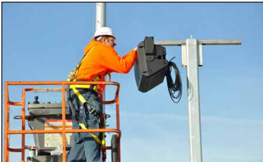
Speaker installation down the leftfield line.
