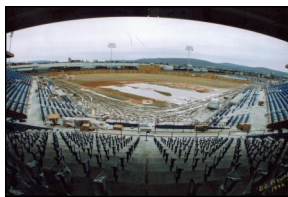
Municipal Stadium under construction in 1992
