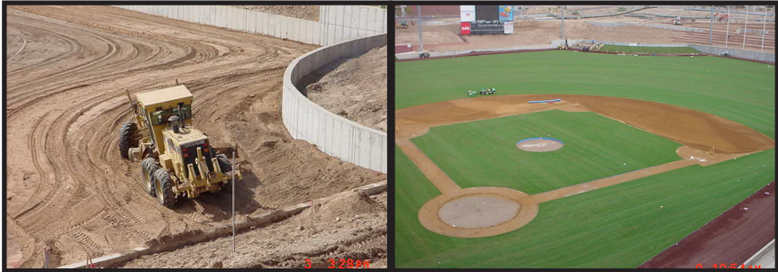
The Hill undergoes construction in mid-2002.
