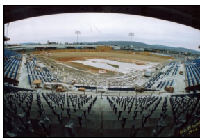
Municipal Stadium under construction in 1992
