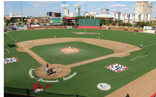
LAWRENCE-DUMONT STADIUM Photo: The Hutchinson News
