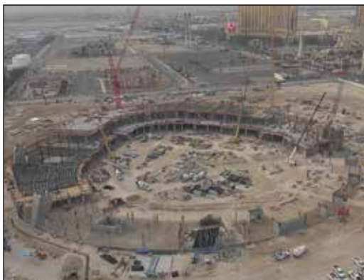
Construction progress of the A's ballpark in Las Vegas as of January 28, 2026. For the latest images, visit ballparkexperience.athletics.com/construction .
